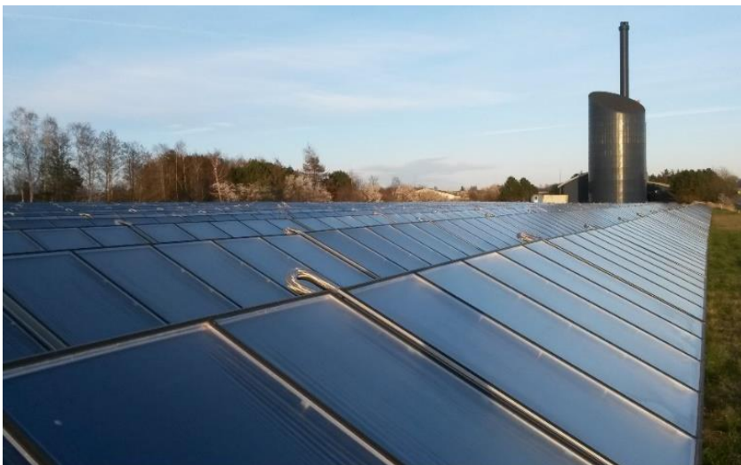
Figure 26. Solar collector field at Helsingø (Denmark) with storage tank and the natural gas fired CHP DH plant in the background [9].
