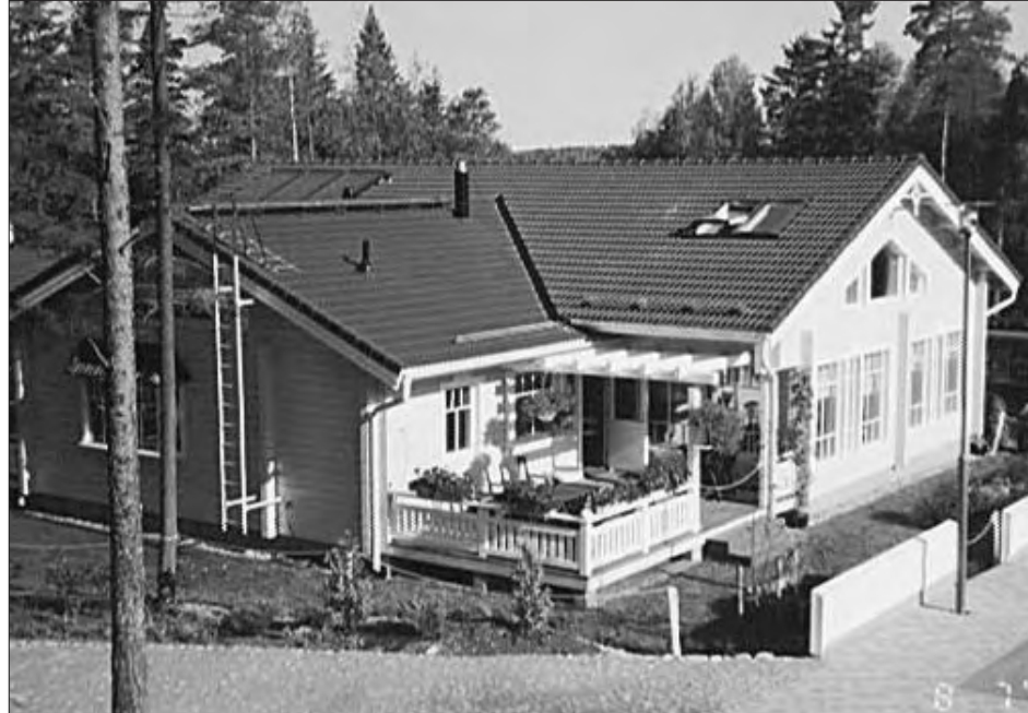
A solar combisystem for a detached house in Finland.
