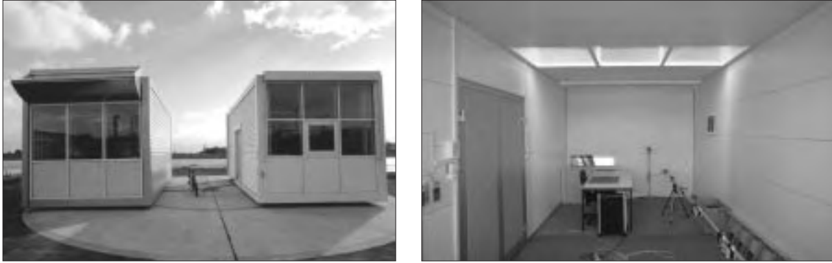
Figure 3. Test facility at LESO, EPFL in Switzerland. Each room has windows on the upper part of the facade, the lower part of the wall being opaque (sill-height is 1.05 m above the interior floor). The system tested in this case is a so-called anidolic ceiling, an innovative system that brings light from the facade to the back of the room.
